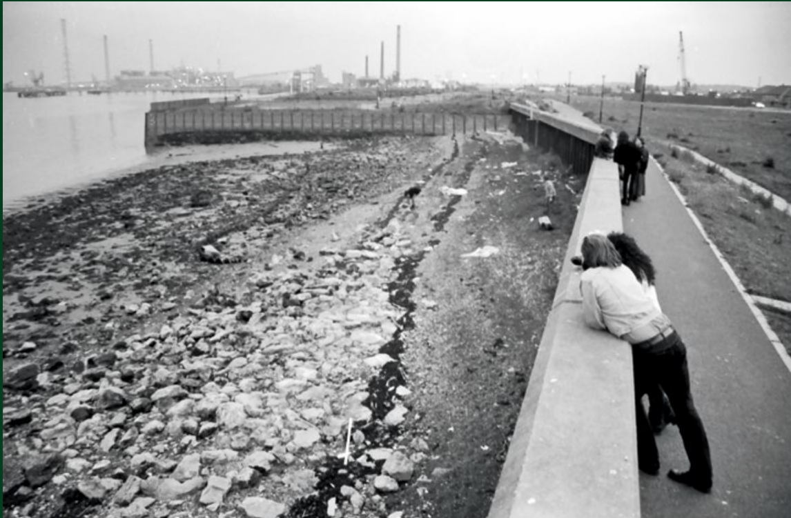
David Kohn, Thames river wall at Thurrock, Essex, 1996
