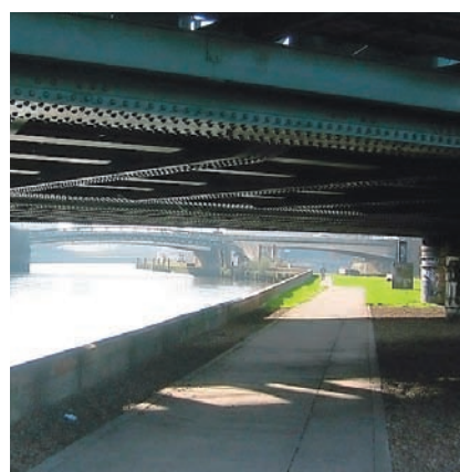
A view along the intended route of 'the Fatwalk' connecting the Olympic site with the Thames. 5th Studio
